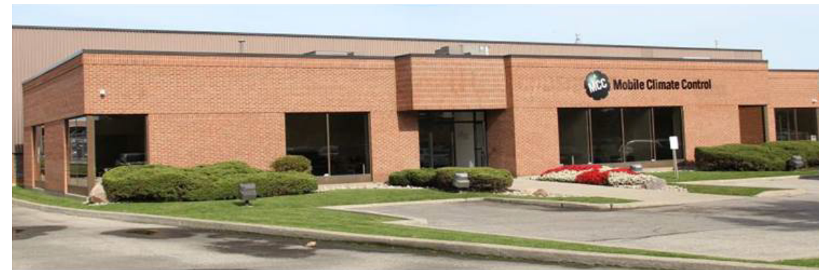
MCC's Microchannel Coil Plant - Mississauga, Ontario
