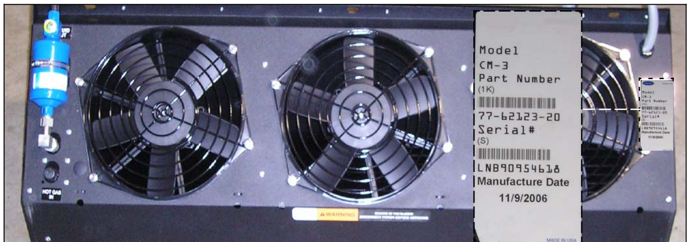
Figure 1-1 Condenser Model CM2/3 - Serial Number Location
