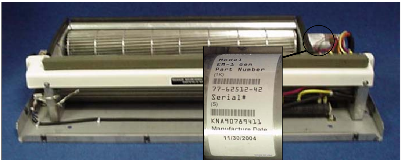
Figure 1-3 GEN 5 Evaporator Model (All) - Serial Number Location
